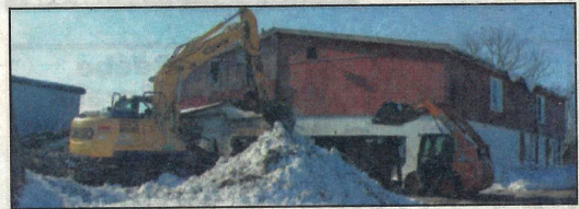
A loader digs into the rear of the building.
